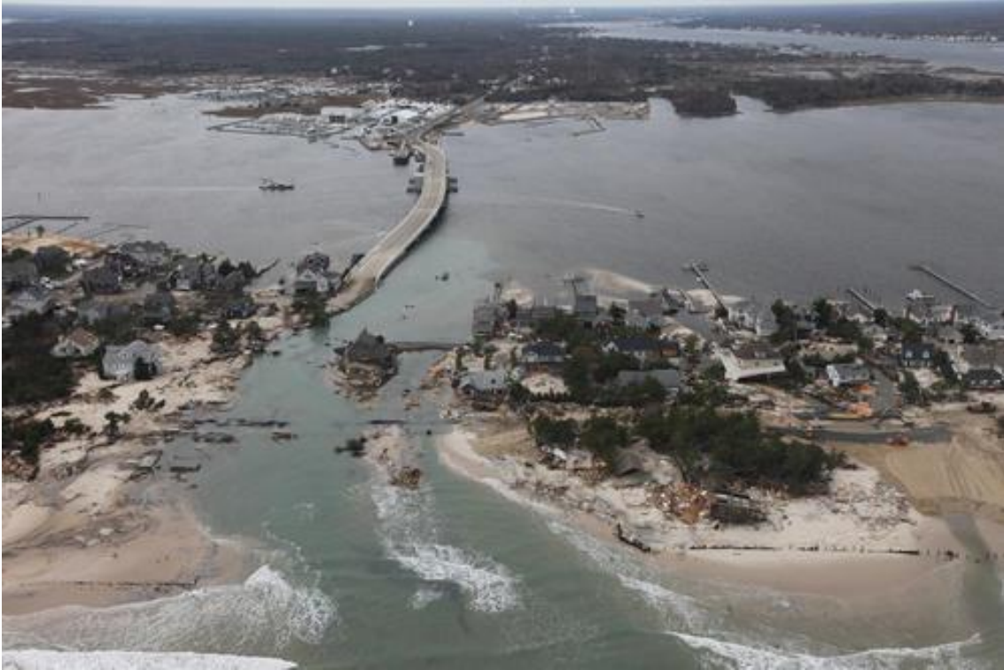
Figure 1.3. Damage from Hurricane Sandy at Mantoloking, NJ. From “Aerial photograph of Hurricane Sandy storm damage at Mantoloking, New Jersey coastline,” United States Geological Survey (2012). Photo by Greg Thompson, USFWS ( https://www.usgs.gov/media/images/aerial-photograph-hurricane-sandy-storm-damage-mantoloking-new-jersey-coastline ). In the public domain.
