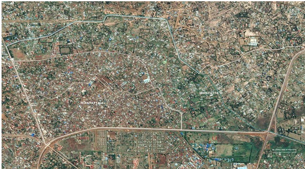
Figure 3.4. Aerial view of Manyatta, an informal settlement in Kisumu, Kenya. Courtesy of the Urban Design Lab at the Earth Institute, Columbia University. Used with permission.
