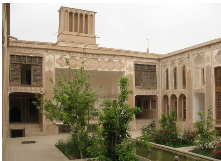
Figure 1.1. Malekzadeh House built during the Qajar dynasty (1794-1925) in Fahadan neighborhood of Yazd, known as city of wind towers, Iran
