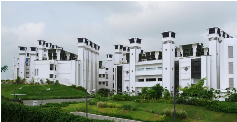
Figure 3.9. Evaporative downdraft wind towers in Torrent Research Center in Ahmadabad, India (Torrent Pharmaceuticals Ltd, n.d.)
