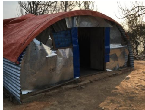
Tarpaulin sheet on roof
