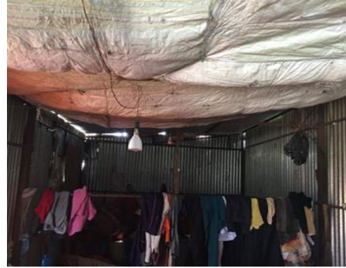
Jute in internal roof
