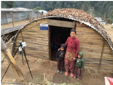
Dry grasses on roof
