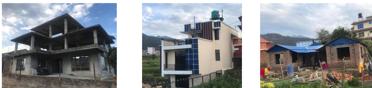
Fig. 1.10 As an example of newly constructed buildings in Lalitpur (Government support and added additional expenses by respondents themselves. Source: Photo taken by author itself).
