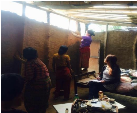
Mud plaster on wall
