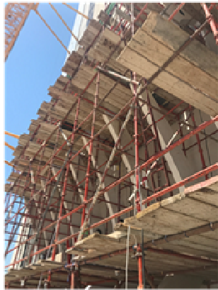
Figure 22. Scaffolding to Support the Canopy
