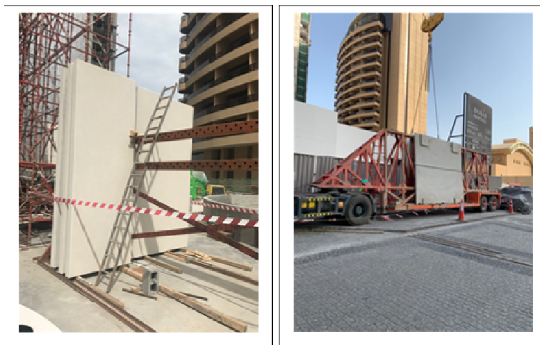
Figures 20 & 21. Precast Panels
