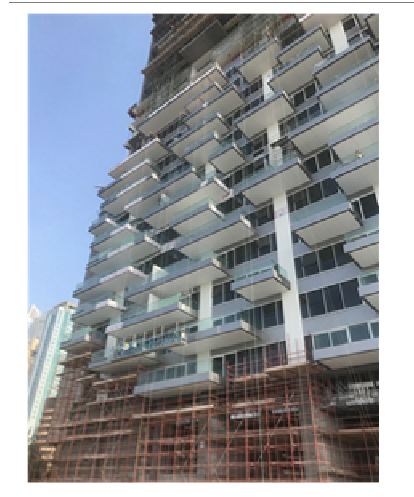
Figure 27. Scaffolding for the Balconies
