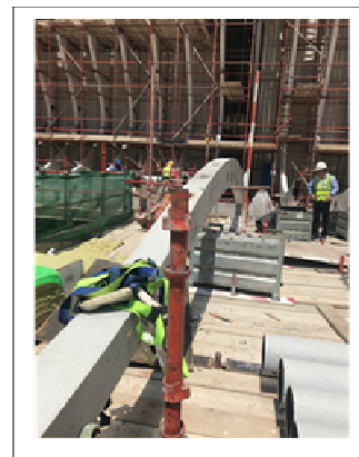
Figure 25. Canopy steel structure
