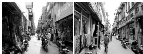
Figure 30. Pictures of Identified Issues along Wool Market Road Based on People’s Perception
