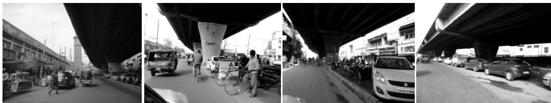
Figure 26. Pictures of Identified Issues along Clock Tower Road Based on People's Perception
