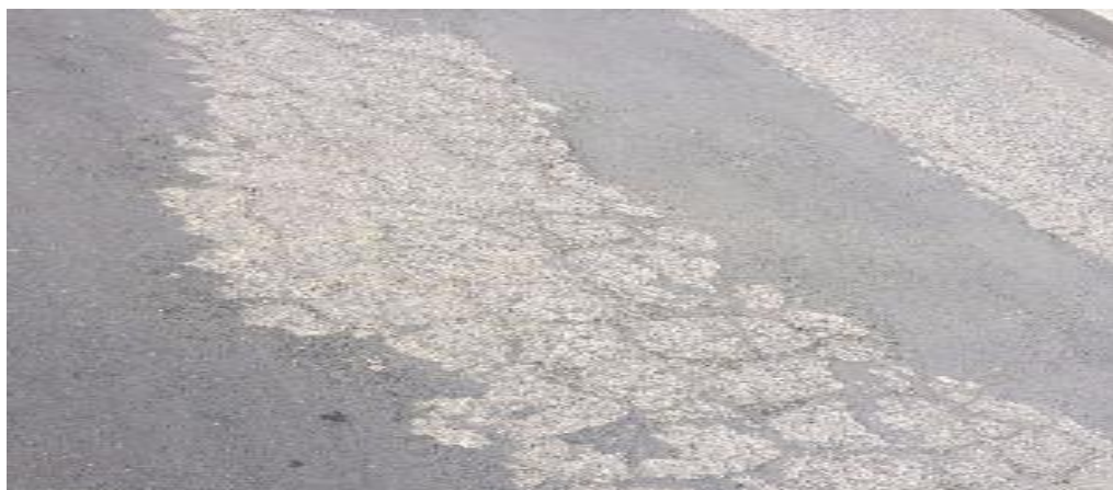
Fig.8: Flexible pavement Patching sample
