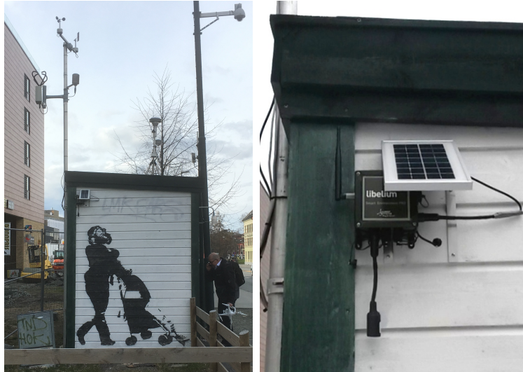
Figure 3: Sensor deployment example: Attachment of basic CO 2 sensor setup next to an official measurement station at a Trondheim major traffic artery.
