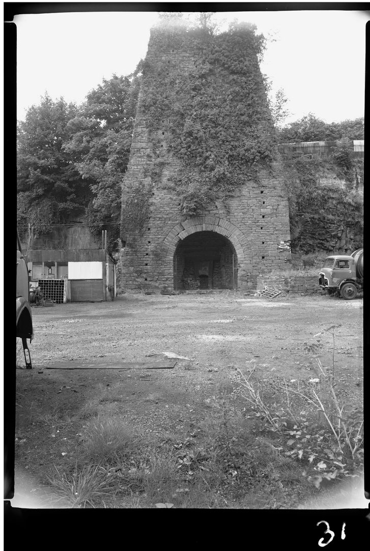
Figure 7.1: One of two surviving blast furnaces at Neath Abbey, South Wales, dating from the Fox-family purchase in 1793. They are set against a rock face for ease of charging, and, at just over 51 and 63 feet tall respectively, are two of the highest masonry blast furnaces ever constructed. Between them stood a Boulton & Watt blowing engine, in front: the casting houses. In nearly a century of operations, the works buried the eponymous monastery in industrial waste; 2024 will mark a century of attempts to excavate it. Neath Abbey ironworks, 1975, photograph taken by John Cornwell, © Amgueddfa Cymru - National Museum Wales.
