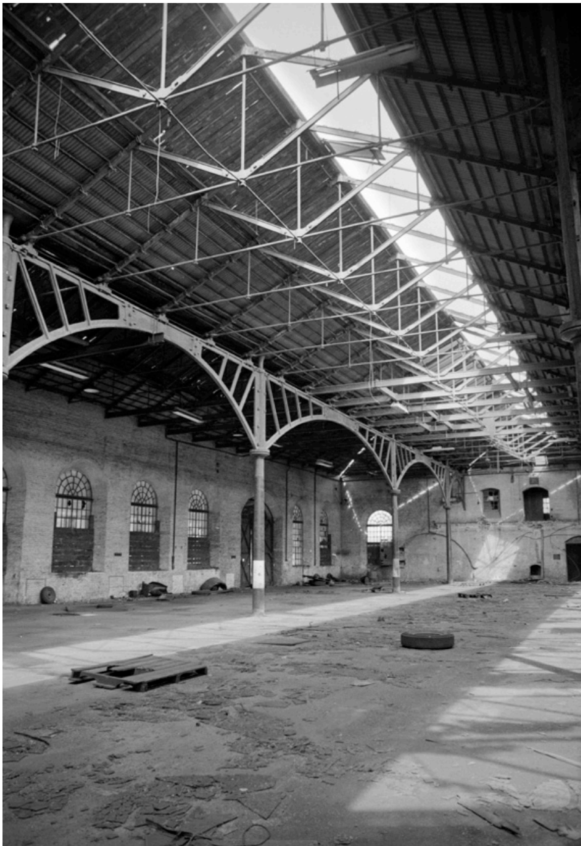
Figure 2.7b: The 1814 iron frame in its original Woolwich setting. The frame was taken down in 1973-4 and re-erected at the Blists Hill site of the Ironbridge Gorge Museum, as shown in Figure 2.7a
