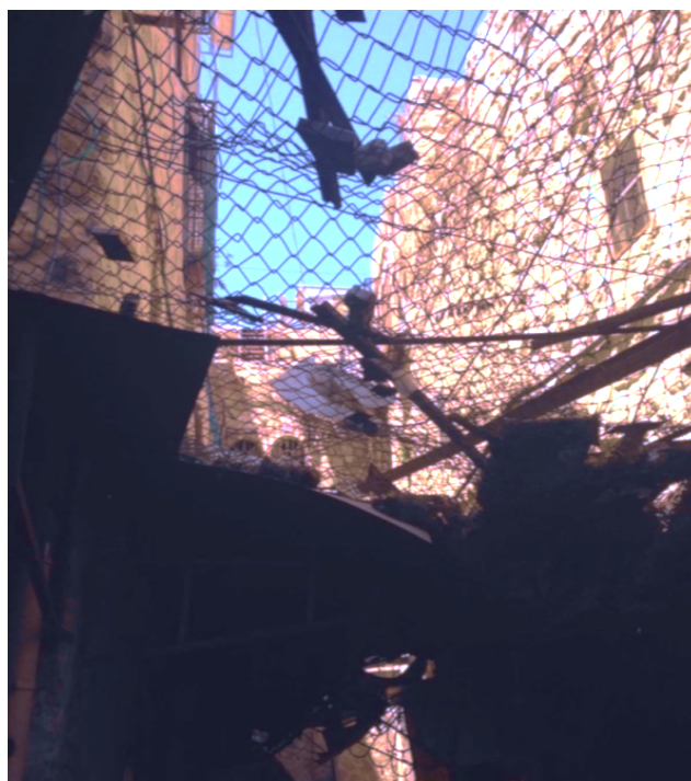
Figure 6 Rubbish dropped on the canopy above the Old City shops
