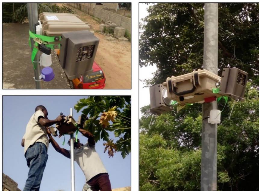
Figure 5 Deployment of the pollution measurement equipment.
