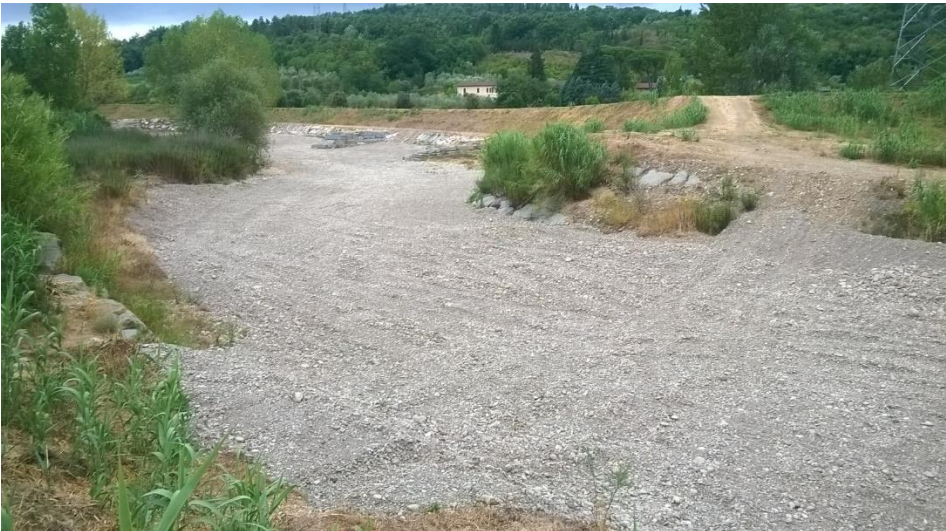
Figure 60 - Final part of Pesa river, close to the Pesa basin outlet (July 2017).
