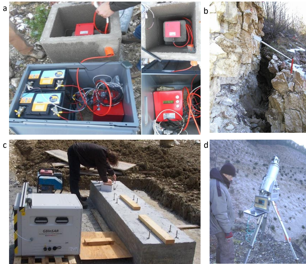
Figure 10. Some examples of instruments employed in Torgiovannetto. Picture a is seismic station (velocimeter sensor) employed in seismic monitoring; picture b is extensometer; picture c is Ground Based Interferometric Synthetic Aperture Radar (GB-InSAR); and picture d is Light Detection and Ranging (LiDAR)
