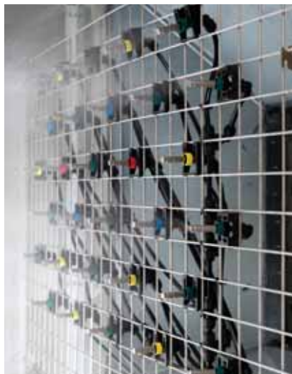
The Condair DL combines spray and evaporative technology, and can deliver 2%RH control.
