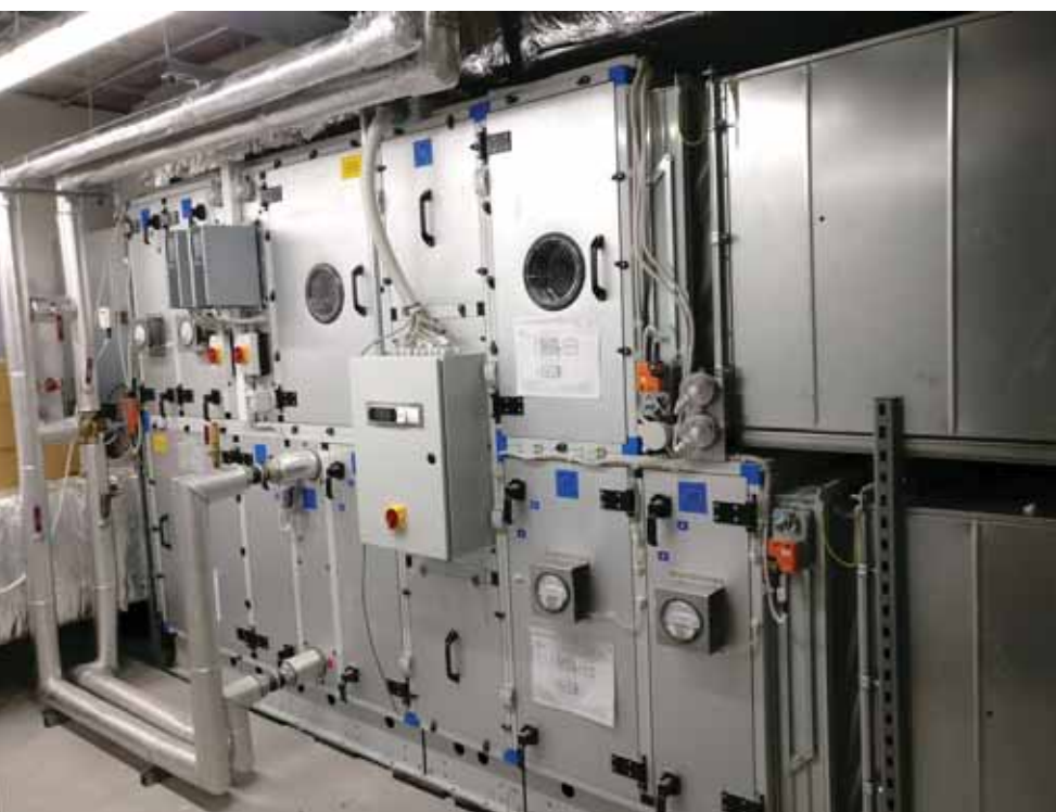
Office fit out in Galway.
