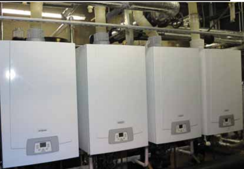
Above: The four commercial Sirius Two WH110 boilers on a cascade frame. Right: St Monica's Nursing Home.
