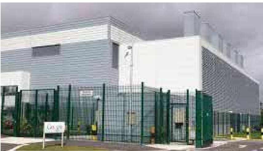
Google's Data Centre in Grangecastle.
