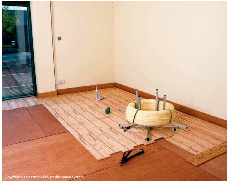
Polytherm's Heattrack low profile panel system.
