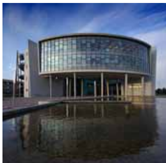
OPW Offices Trim
