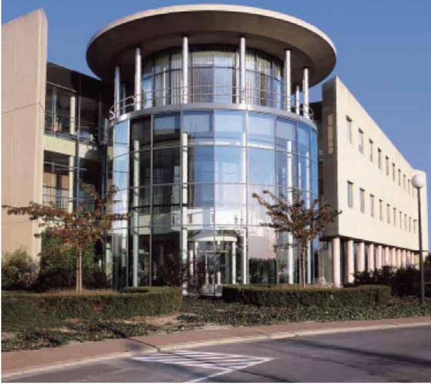
The Daikin Industries European headquarters in Ostend, Belgium
