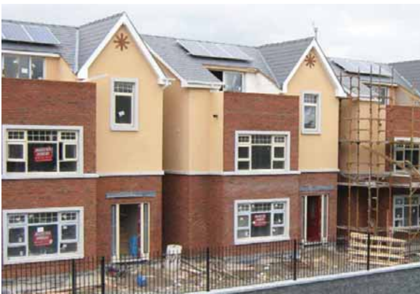
The Dimplex solution at Cherangani resulted in Part L compliance, and an A2 BER rating
