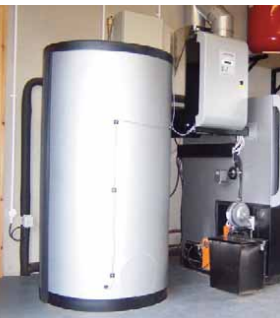
Figure 5 – Typical domestic biomass boiler with fuel store (wreep.homestead.com, 2013)
