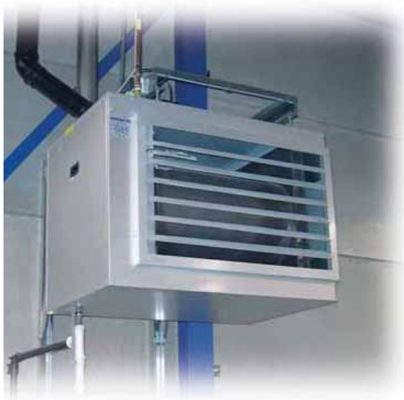
Mark GS+ high efficiency warm air heater with axial fan.
