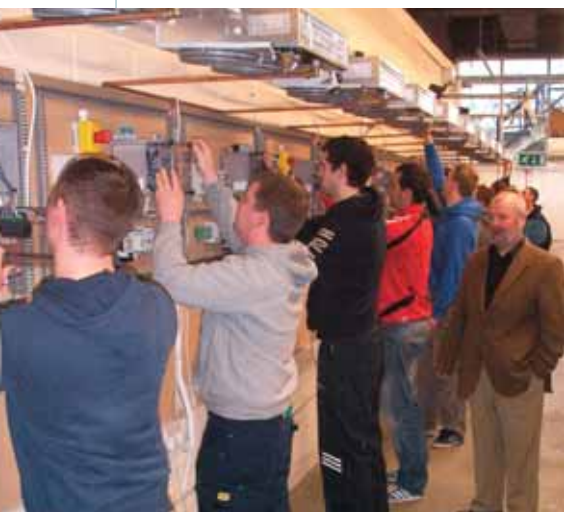
Lecturer Tony O'Brien overseeing work on the installation.
