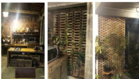
Gambar 17. Dinding bata ekspose didapur dan kamar mandi lantai 1 (Survey Lapangan, 2019)
