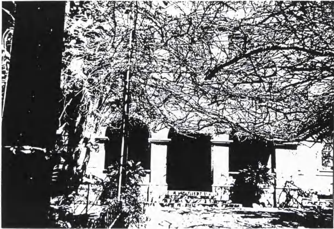
Figure 48: Gibraltar Courts, entrance
