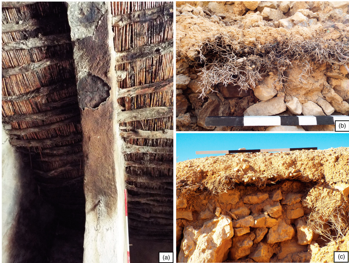
Figure 3. Al Ma'tan Roofs: (a) Typical roof construction showing supporting Juniper beams ( Juniper phoenicea ) with reeds ( Phragmites australis ), as seen in Building 1. (b): roof construction showing 'bilan' ( Sarcopoterium spinosum ) on top of the reeds, Building 1. (c) roof construction showing thick layer of sediment with stony inclusions above the 'bilan' and the reeds.
