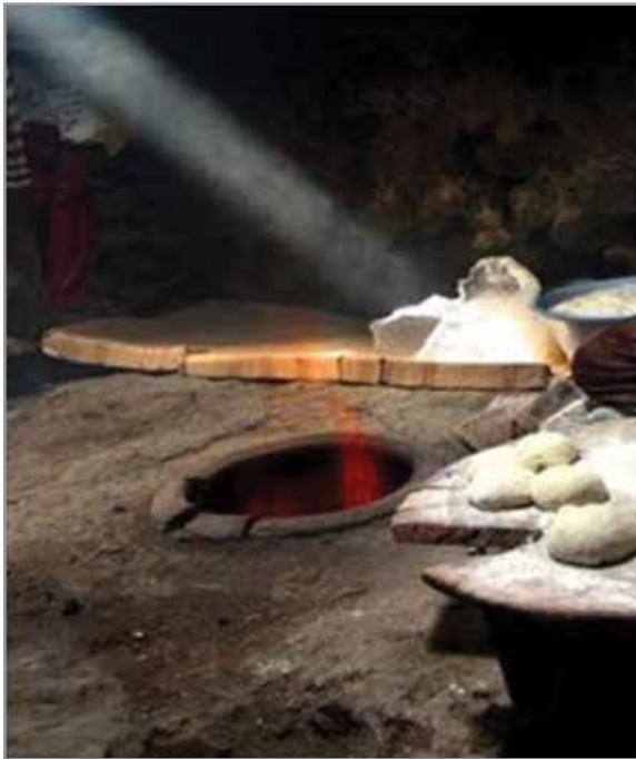
Figure 1. Lack of chimney and poor smoke ventilation.
