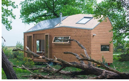
Şekil 3.10 Walden Studios – Dimka Wintzel Tiny House – Solar Enerji Panelleri (Archdaily, 2019)
