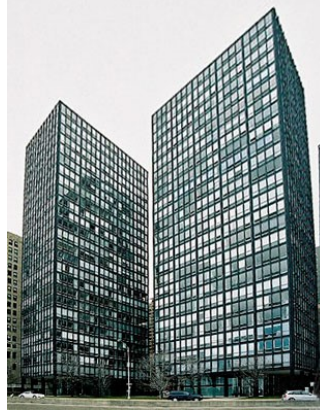
Şekil 1.9 Twin Towers, Mies van der Rohe, Chicago (1928-1931) (The High Rise Pages, 2018)
