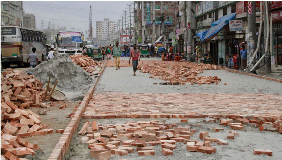
Figure 5. Road construction using Bangla bricks. Credit: Author.
