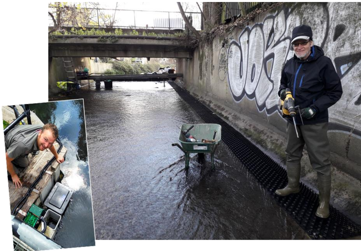
Figure 10 Installing eel migration tiles at Garratt Lane and (inset) an eel monitoring box at MHP
