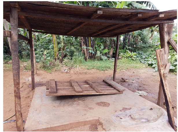
FIGURE 3 | A rural slaughter slab with a pole mounted roof and a wooden pallet. Photo: Linda Waldman.
