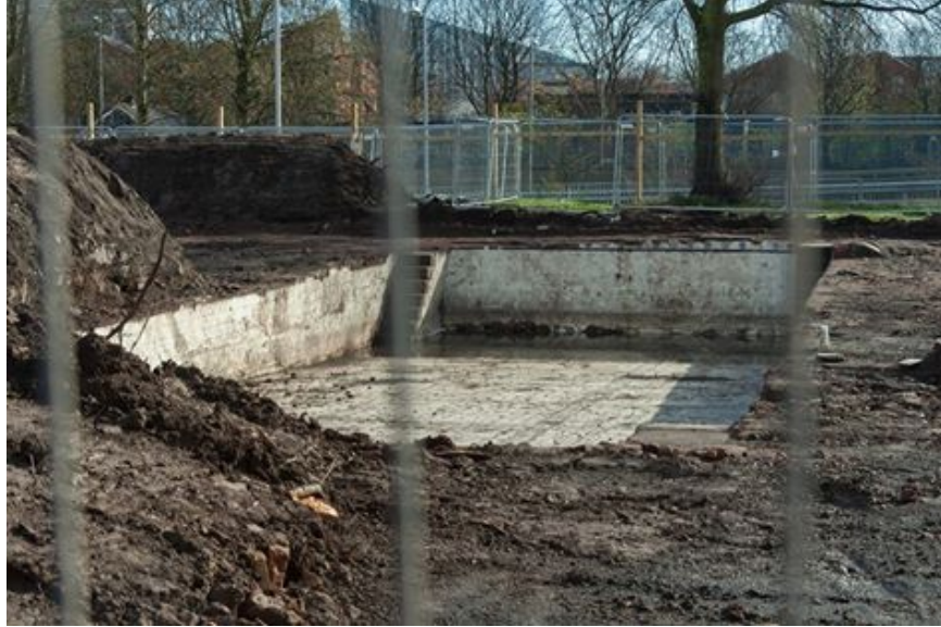
Image 24: Leaf Street baths during construction (Wilson, 2016)
