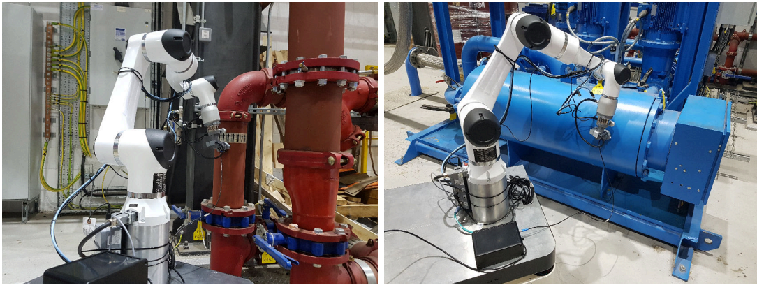
Fig. 1. Robotic non-destructive tank and pipe inspection using a mobile robot. The operator can inspect parts of the asset remotely and without decommissioning the asset for the duration of the inspection.
