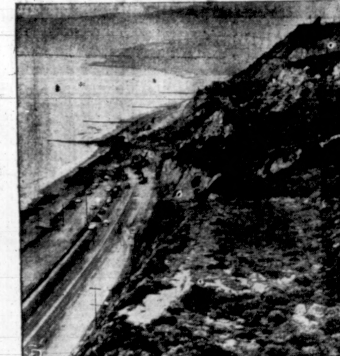
FOUR-LANE ocean highway near Santa Monica, Calif., is shown buried under an estimated 50,000 tons of earth following a sudden landslide from the cliff. (International Soundphoto)
