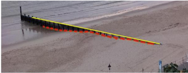
Figure 5: Sand level detection at Bournemouth with sand level (red line) identified and top of groyne highlighted (yellow line).
