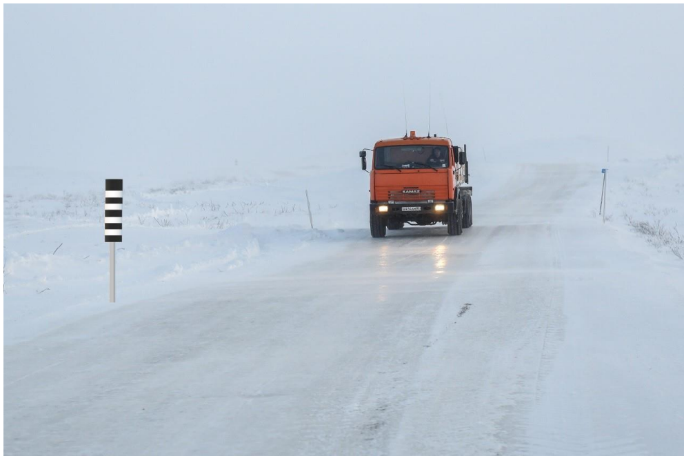
Figure 9 - An example of installing a marker on a winter road
