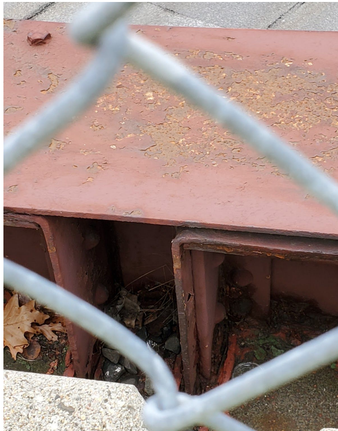
Photo 12: Connection of girders at center of bridge.
