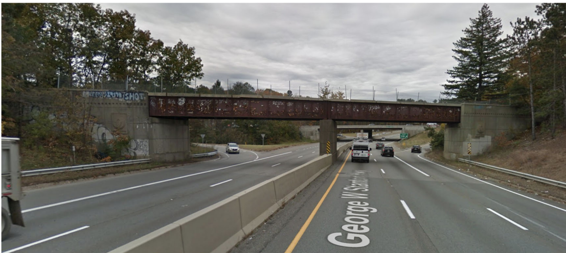
Figure 4: Framingham and Worcester Railroad Bridge Over Route 2 in Leominster (Google Maps, 2019)
