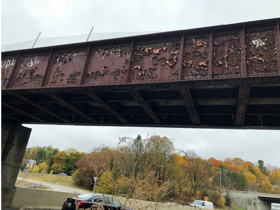
Photo 3: Underside of bridge from shoulder of Route 2, looking southwest.
