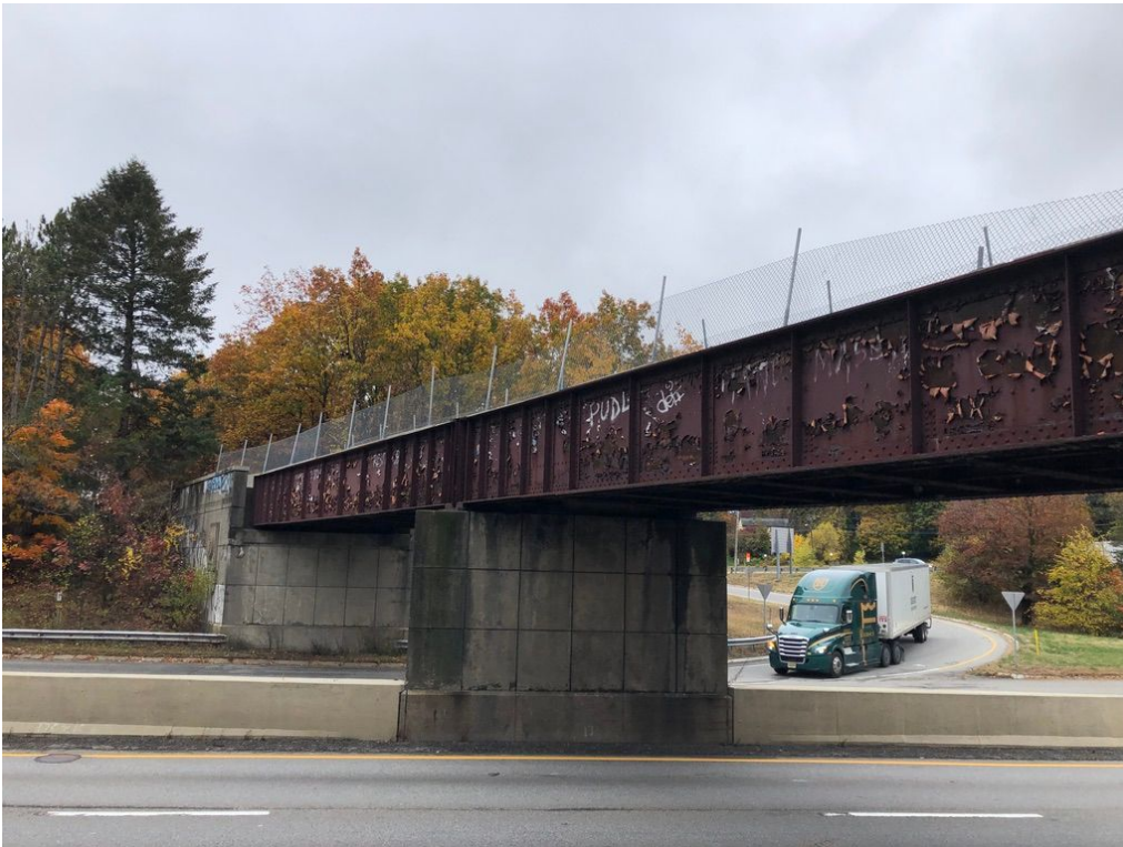
Photo 2: Looking southwest, view of bridge from shoulder of Route 2.
