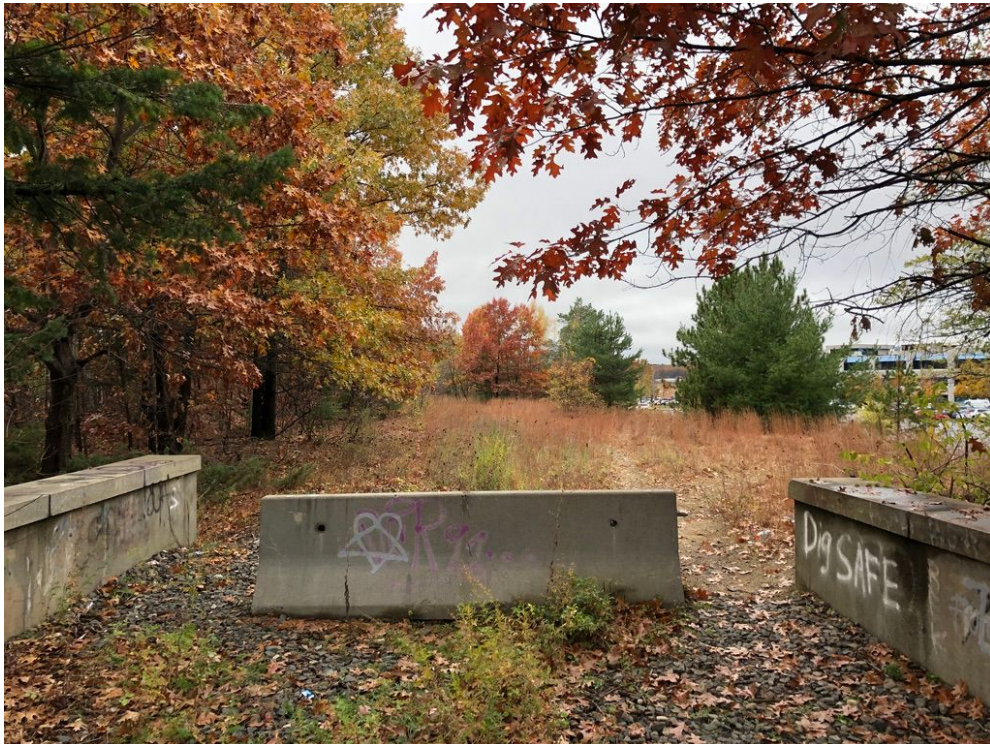
Photo 8: Path leading to bridge, looking north.
