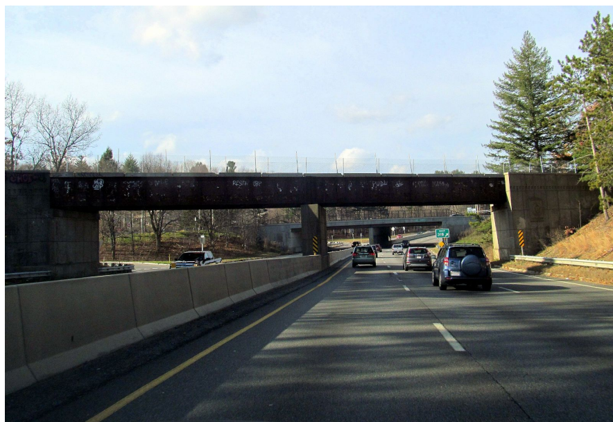
Fig 1: Framingham and Worcester Railroad Bridge Over Route 2 in Leominster (Pi.1415926535, 2015)
