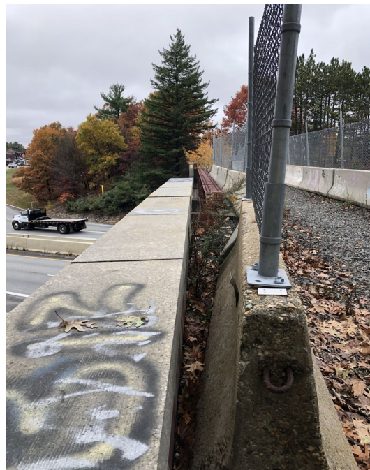
Figure 15: Existing Bridge Railing on West Side of Bridge (Morrison Ouellette, 2019)
