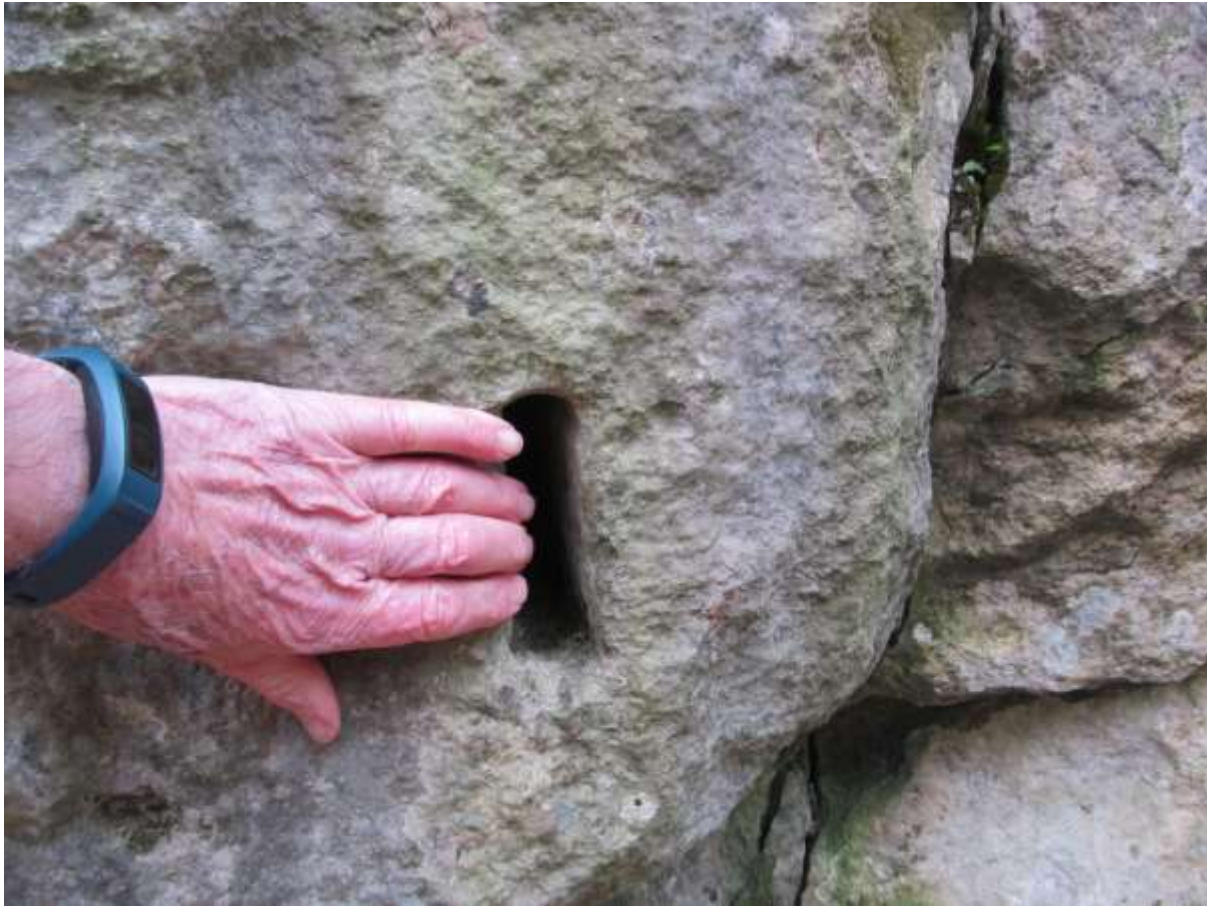
Figure 7. Lewis bolt-hole from Brown's Folly. The length is 10 cm, but that increases inwards, width 2.5 cm and depth 12 cm.
