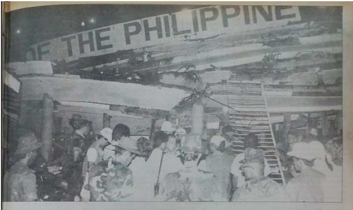
Photo No. 22.3: A closer of the collapsed CCP Building
