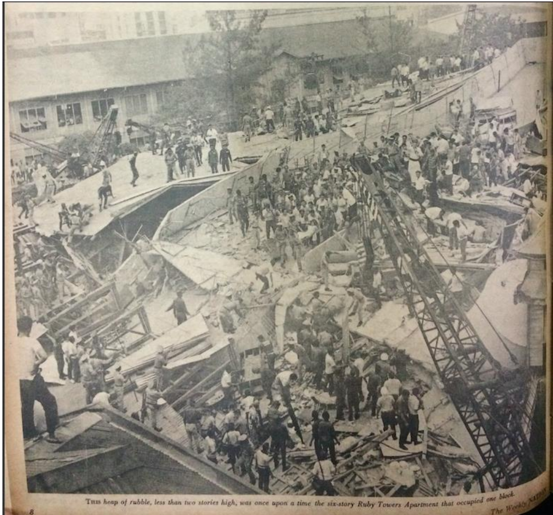
Photo No. 11 The Collapsed Ruby Tower after the 02 August 1968 Earthquake 1172
