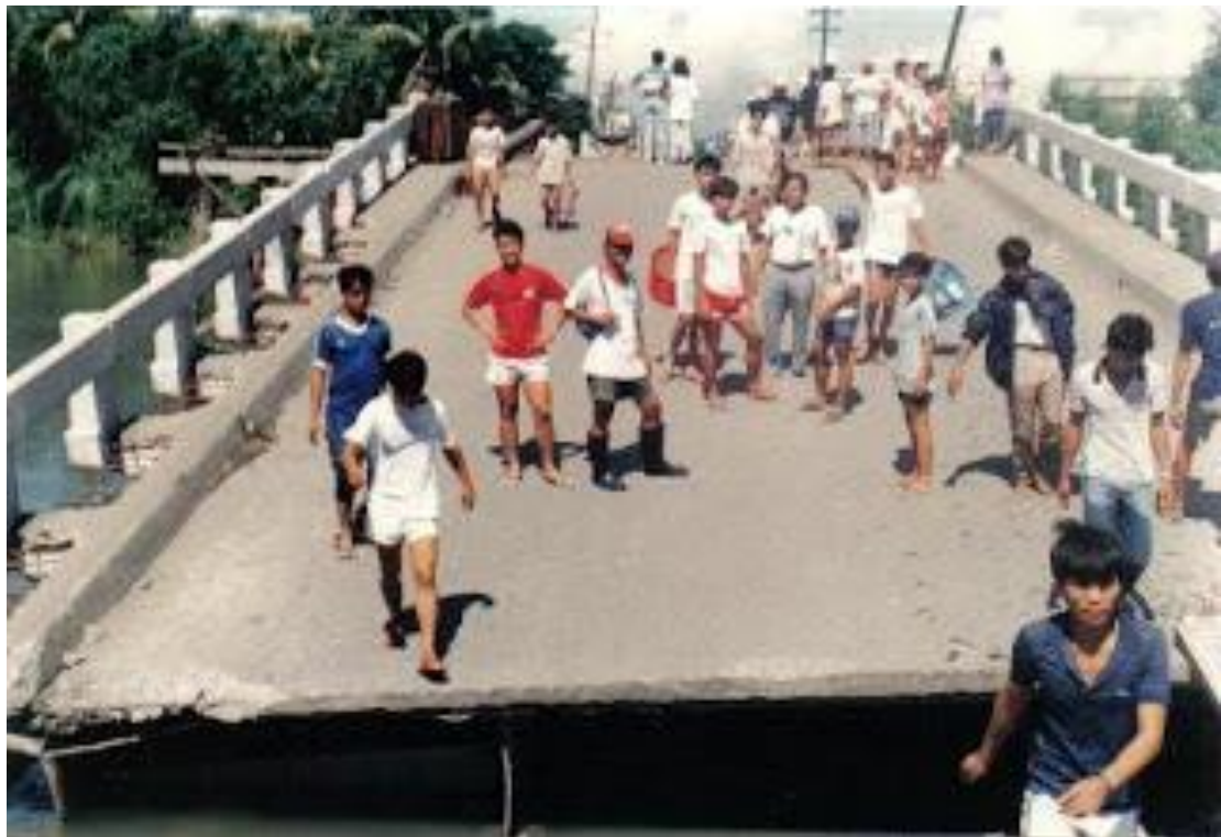
Photo No. 23.4: A photo showing a destroyed bridge
