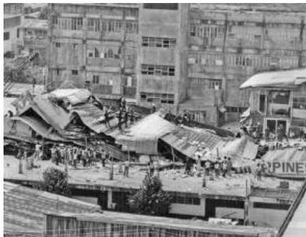
Photo No. 22.1: Aerial view of the collapsed CCP Building
