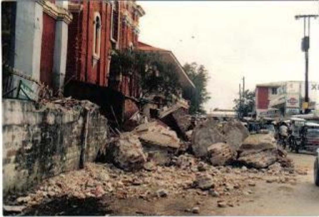
Photo No. 23.3: A photo showing the damaged buildings in Dagupan
