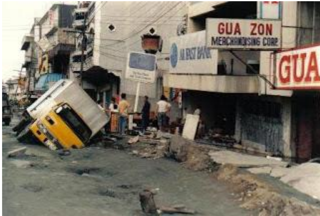
Photo No. 23.1: A photo showing vehicles eaten up by roads that suffered liquefaction
