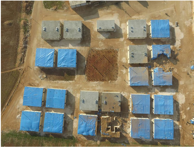
Fig. 6 The destruction and bombing damages in the pilot project, Ariel photo. Source: Binaa for development (2016)
