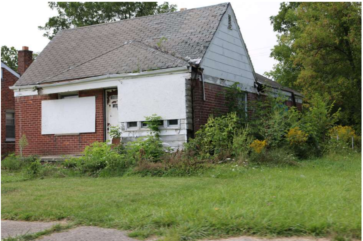
Figure 29 Abandoned house with boarded up windows, August, 2016
