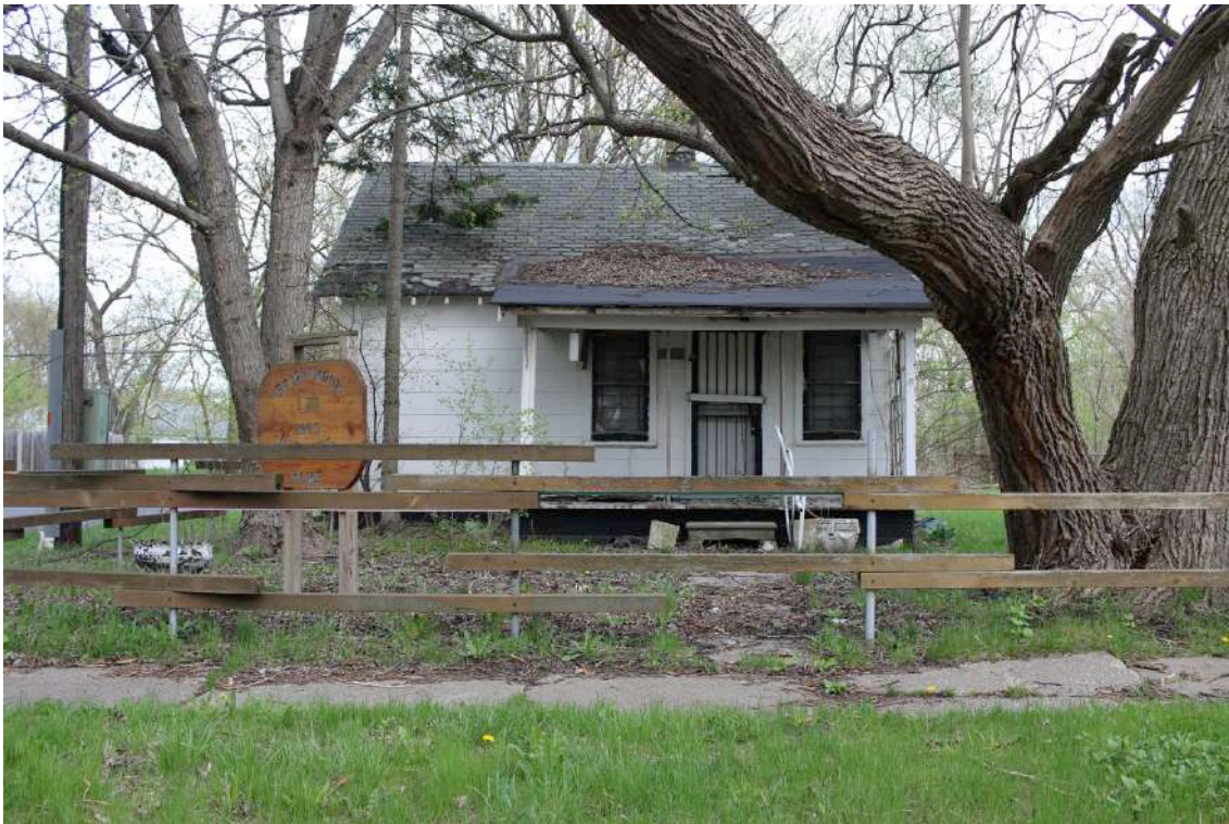
Figure 27 15378 Lamphere Street. One of the few existing original 'Taylor Homes' constructed for the Brightmoor neighbourhood. April, 2018
