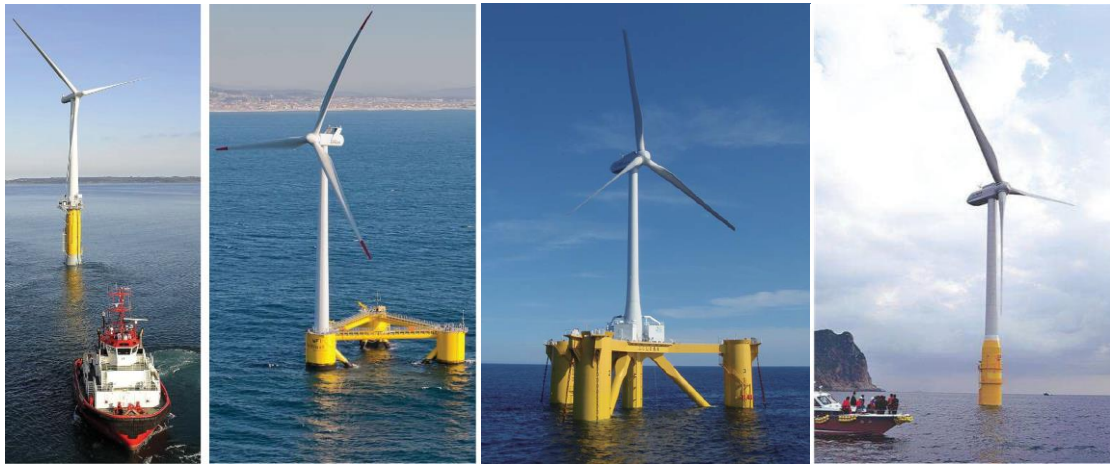
Figure 5: Prototypes of floating wind turbines (from left: a) Hywind (Statoil, 2014); b) WindFloat (PrinciplePower, 2014); c) Fukushima semi-submersible (FOWC, 2013); d) GOTO spar (GOTO-FOWT-Website, 2014))
