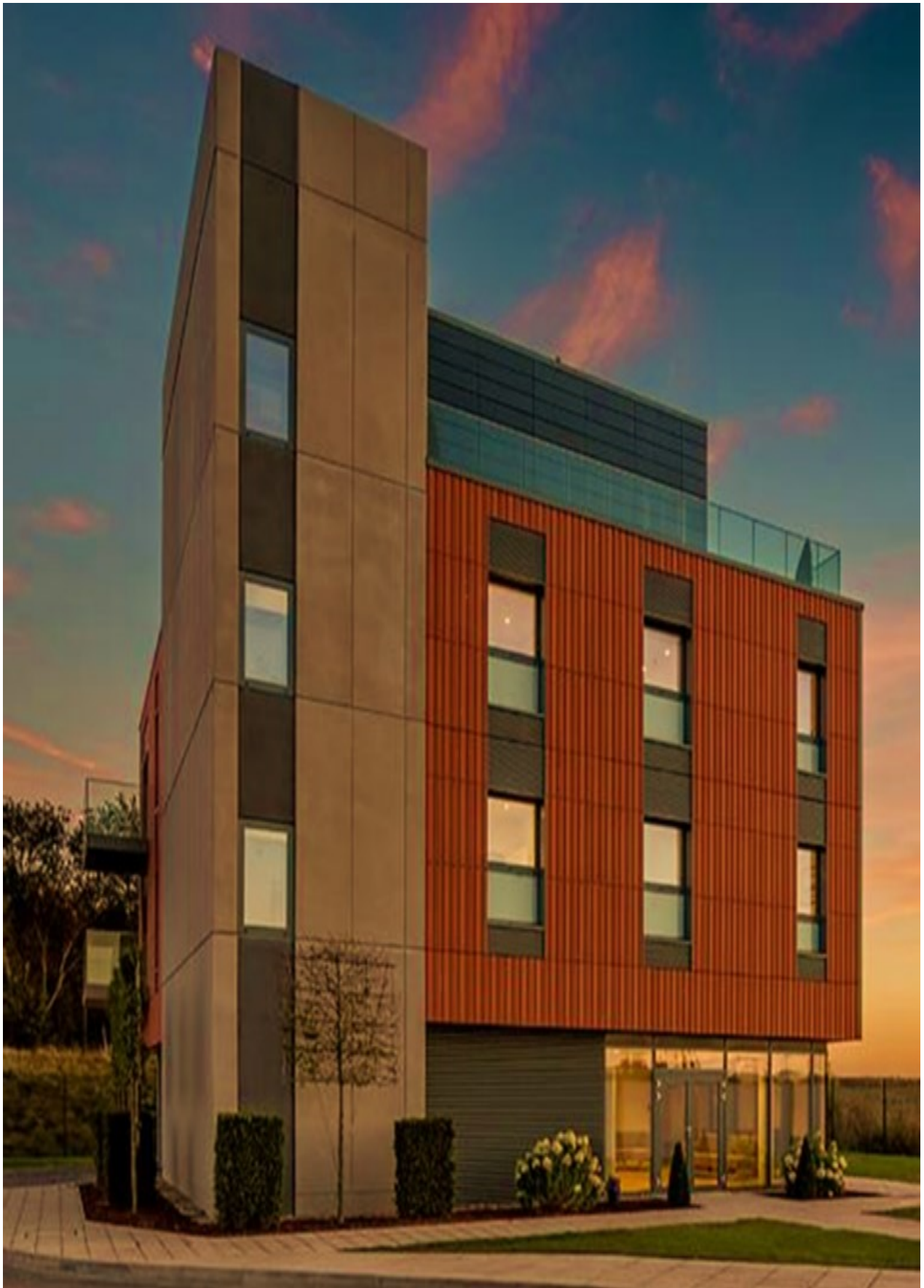
Figure 6.1. A generic apartment building (Source: Laing O'Rourke)
