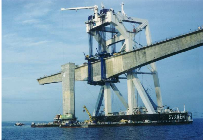
Figure 3 – HLV Svanen Placing a Main Bridge Span
