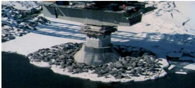
Figure 12 – Armour Stone Scour Pad at Shallow Water Approach Pier (photo by Boily)
