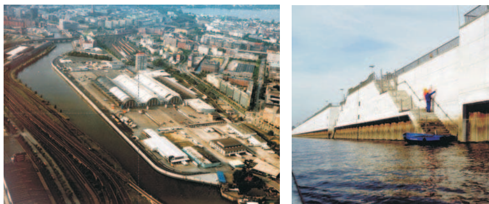
Fig. 6: Public storm surge protection wall at Großmarkt in Hamburg (left: aerial view; right: wall as seen from the water) (photos: LSBG, 2003)
