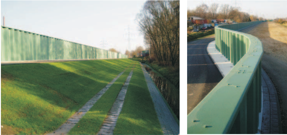
Fig. 7: Public storm surge protection: Bostelbeker main dike (left, length: 770 m) and sheet pile wall section at Bostelbeker main dike (right) (photos: HPA, 2007)
