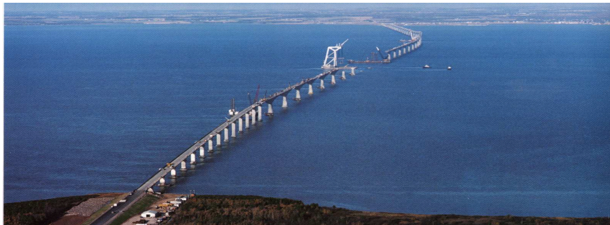
Figure 3 – The Confederation Bridge (photo by Boily)
