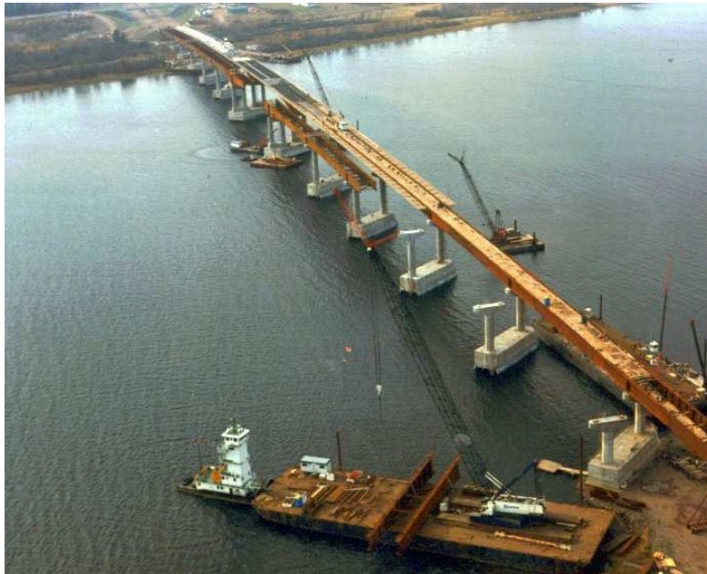
Figure 1 – The St. John River Bridge
