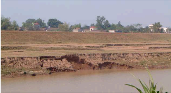
Figure 13. Example of a sliding due to toe scour in an outer bend
