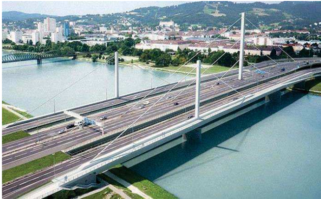
Figure 2: Voest-bridge with additional side-bridges 6; project by consortium: Bernard Ingenieure, RWT plus ZT GmbH and Solid architecture.
