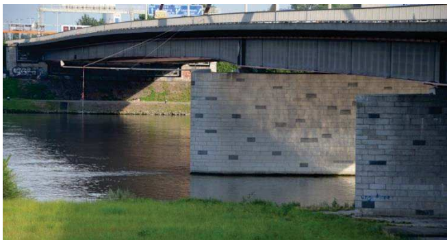
Figure 3: Voest-bridge with existing bridge piers
