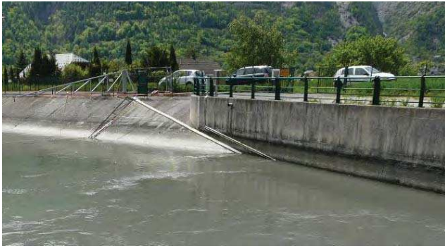
Fig. 3 Measuring flow and water level using a radar sensor at the downstream extremity of the channel
