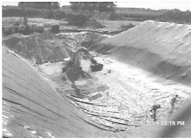
Figure 4: Filling the basin with sand and build-up of the clay levee
