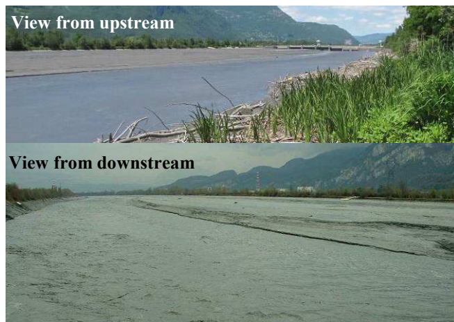
Figure 2. St Egrève reservoir during a flushing event.
